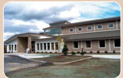
The exterior work on Speare Memorial at Boulder Point is nearly complete. Photo taken on October 6.
